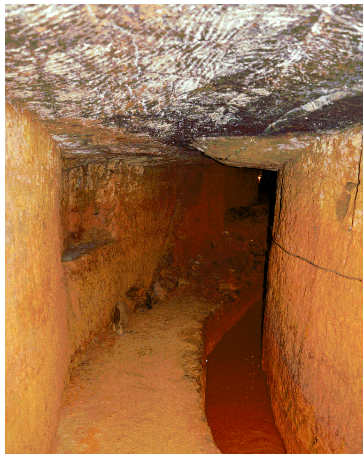
Minamizawa Drainage Tunnel took six years to cut with only a slight difference of at most 1 m along for the 922m length.
